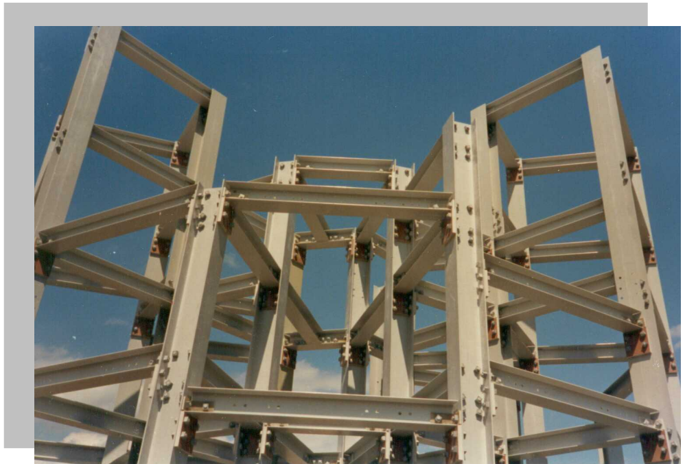
Nuclear test tower constructed using Pultex® Standard Structural Profiles
